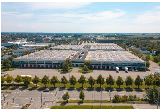
BMK location at Technology Campus Augsburg, 86199 Augsburg picture source: Bernd Jaufmann
